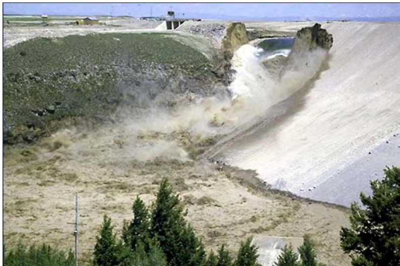
Failure of Teton Dam (Idaho) from seepage (1976)
