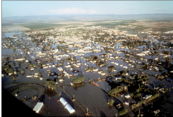
Flooding caused by the failure of Teton Dam in eastern Idaho as it was filling for the first time (1976); 14 people died ( waterarchives.org )
